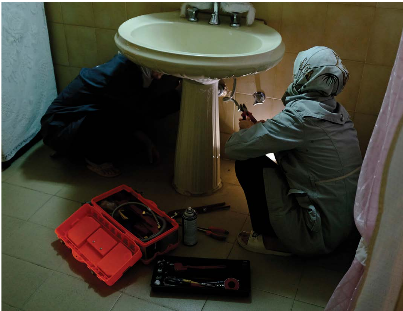
Above: Safa'a (right) is Jordanian, Hajar (left) is Syrian. They work together, providing plumbing services in Irbid, Jordan. Timea Fauszt/IRC
